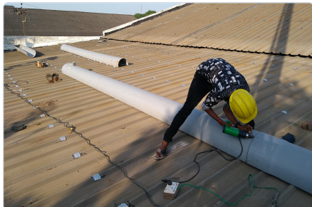
Industrial Shed Rain Gutters
